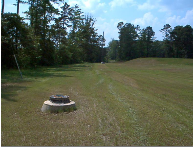
Figure 4: 2000 Bond Projects - Sewer Line Near U. S. 58 Bypass
