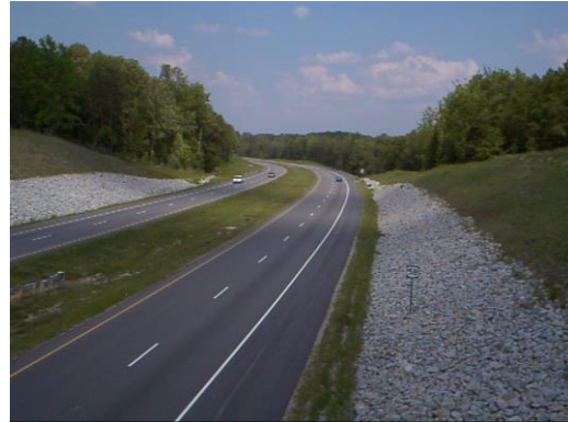
Figure 5: U. S. 58 Bypass as seen from Goode's Ferry Road
